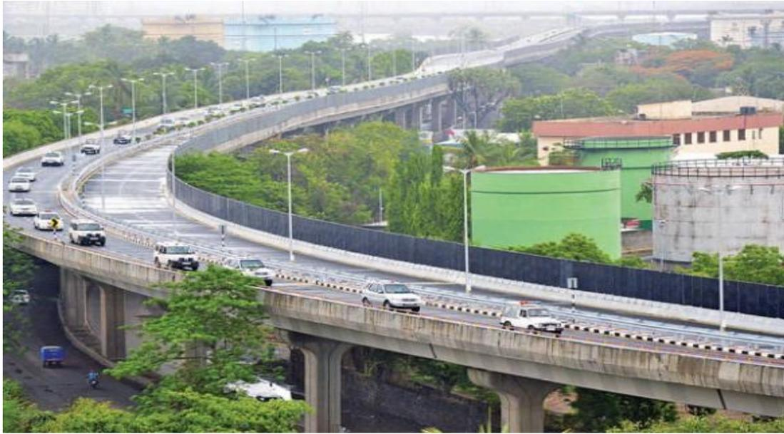
**The controlled-access freeway** is 16.8 km long Eastern Freeway comprising of three segments, one of the twin tunnels, 13 km elevated road and Ghatkopar-Mankhurd Link Road. Eastern Freeway reduces travel time between South Mumbai and the Eastern Suburbs and ranked as one of the Outstanding Infrastructure Projects of the Country.
